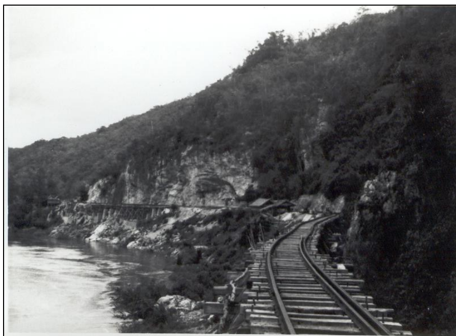
Wampo South Viaduct looking up river (1950) 7
