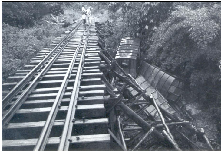
Wrecked rolling stock adjacent to repaired section of railway (1945) 5
